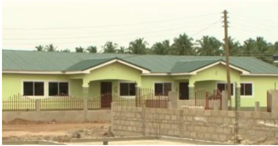
GHS' Willow Court under construction
