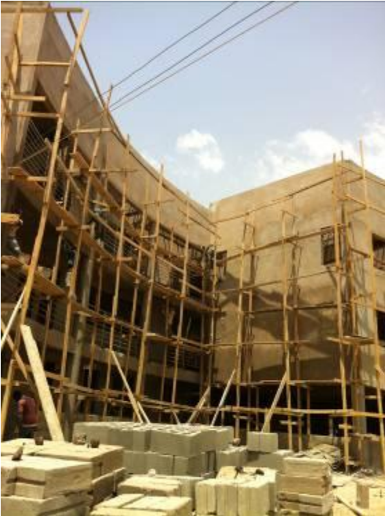
The Dome site under construction in H1 2013
