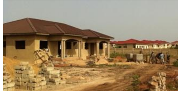
Redrow's Second Site Under Construction
