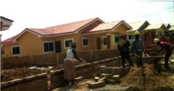
GHS Construction in Pokuase Accra
